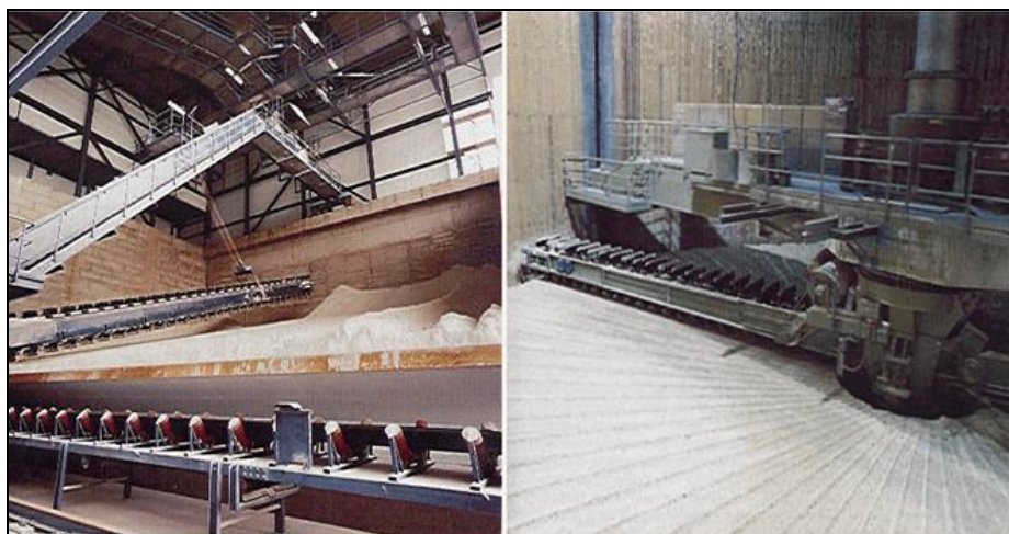
Figure 4.23: Closed gypsum storage facilities [94, Umwelt + Technik, 2000]
